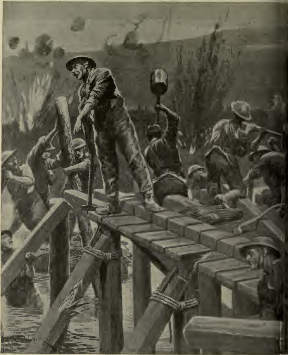
British Engineers building a Bridge
